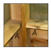
Once a location has been determined carefully unpack the panel sections. The corners of each panel are market with a letter. There are two panel edges that have the letter "A". The 2 A's go together and form a corner. A helper may be needed to hold the panels together until some screws are holding them together Each corner joint should have 3-4 screws installed as shown
