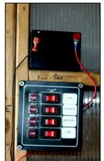
Install the battery on the shelf above the switch panel and connect the two leads, red-to-red, and black-to-black. Check to see that the green cable is tight and wrapped around all the pulleys as shown on the right. Check to see that the turnbuckle on the traveling car is free to move. The car should be at or near the bottom of the track – this is the
