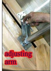
out thru the slot between the roof and the gable end a few inches and position it against the upper swing arm over the door. Slide the other end onto the 4" long tube of the long arm as far as it will go. You should now be able to slide the opposite end (over the doorway) onto
