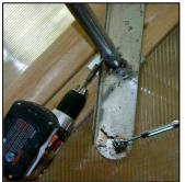
Make sure both ends of the roof are closed. Make sure the torque tube is positioned so the adjusting arm and adjusting bolt (entrance end) can be moved freely and are lined up squarely. Install 2 Tek screws in the torque tube to secure it to the 4" sleeve in the long arm. There may be a hole predrilled in the torque tube. Use them and the Tek screws will drill thru the inner sleeve.
