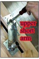
inside and install the hinge arms. The top of the roof will have to be lifted into position over the studs at the gable end peaks. It will not slide fully into place without lifting the top. Now install the swing arms as shown to hold the roof in place. The two arms without large tubes welded onto them are the lower arms. The studs they slide over are of two different lengths and the short small tube goes over the longer stud. The long arm goes over the opening mechanism
